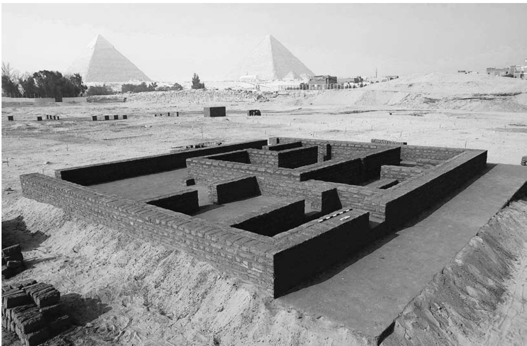
Figure 13. The completed reconstruction of the Eastern Town House built on top of a thick layer of sand over the ancient house. View to the northwest
